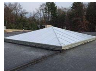
New Skylight - Exterior
