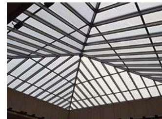
New Skylight - Interior
