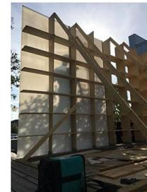
The north gridwall of the MODESTEhouse is clad in 25mm Clear Triplewall Polycarbonate Panels filled with Lumira® aerogel. Multifunctional, the aerogel-filled polycarbonate panels fill the tiny home with beautiful, diffused light, providing privacy while reducing the need for artificial light. Because aerogel particles inhibit heat transfer, the inhabitants of this tiny home will benefit from energy cost savings as well as occupant comfort.
