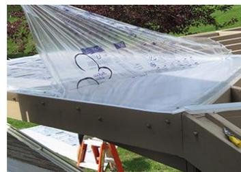
Polycarbonate sheets come covered with a protective masking film. The film indicates the UV protected side which needs to face towards the sun. This protective masking should remain in place to protect the sheet during installation but be removed immediately after the sheet is installed.
