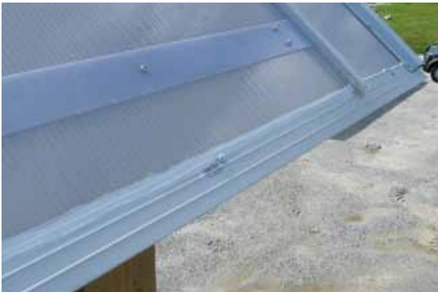
Attach optional extruded U channel or metal drip edge flashing to drip edge
