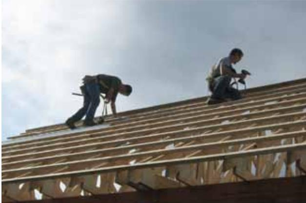
Once building has been framed to code and horizontal purlins installed, install ridge cap to framed building
