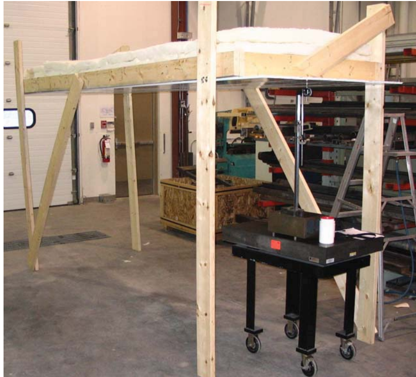
Figure 2 – Panels Loaded with Insulation
