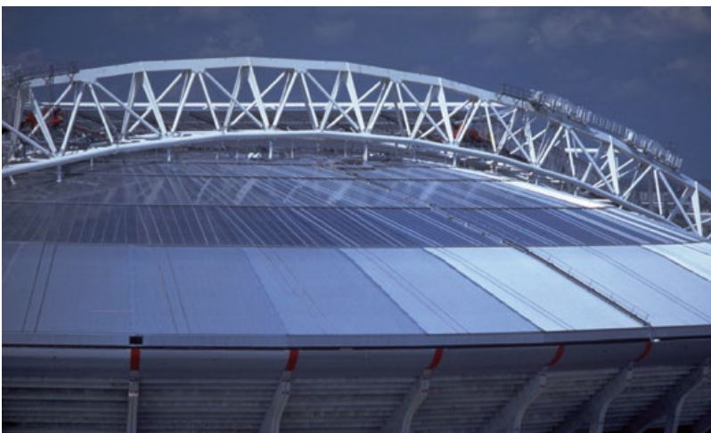
Amsterdam Arena in Amsterdam, the Netherlands is Europe's first stadium with a sliding roof, made from LEXAN™ THERMOCLEAR™ transparent sheet. 20.000 m 2 - The sliding roof was necessary to allow events to be staged regardless of the weather.
