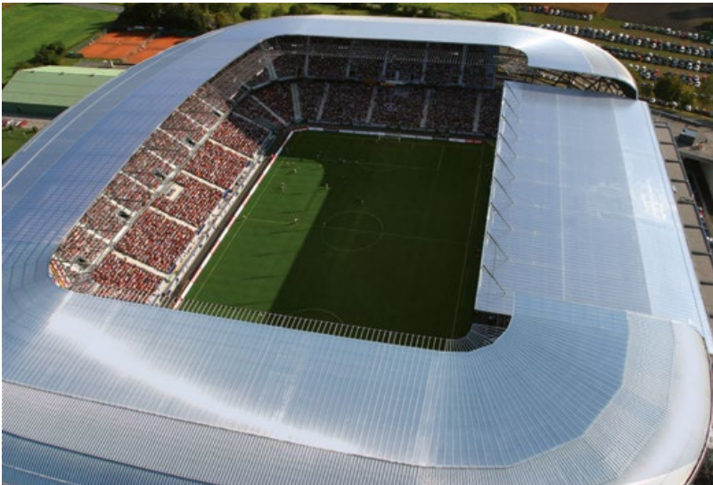
Wörthersee Stadium Roofing. Roof is made of transparent LEXAN™ THERMOCLEAR™16 mm sheet.
