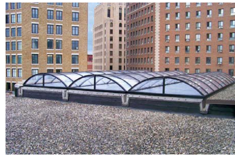
Iona County Court House Wasco, Lumira-filled skylight
