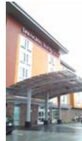
The first impression of any building is the entry. Defining the main entrance of the Springhill Suites is a spectacular exposed steel and standing seam canopy. The structural steel members of the arched canopy are covered with the LEXAPANEL™ 20mm 5-wall X-structure polycarbonate standing seam system. Bronze colored LEXAN™ multiwall polycarbonate sheets were used to filter the glare of the sun and provide maximum shading over the southern exposed front entrance.
