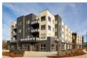
The 951 apartment units feature many great amenities including private balconies. LEXAN™ 16mm polycarbonate panels were used for the balcony railings and the overhead canopies. A combination of Clear and
