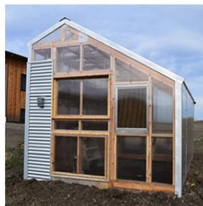
Other key elements in this passive solar greenhouse design include: a heater for when the sun goes down, an exhaust fan to control the heat, a circulation fan to keep the air inside the PSG moving, and strategically placed vents to create
