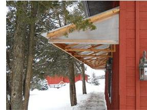
Even though polycarbonate panels offer outstanding snow load capabilities, wet snow can be very heavy.
