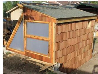
Compared to glass, multiwall polycarbonate panels are lightweight, flexible, and easier to work with. "It was like working with plywood. The panels were very easy to cut. Polycarbonate is also less expensive than glass."
