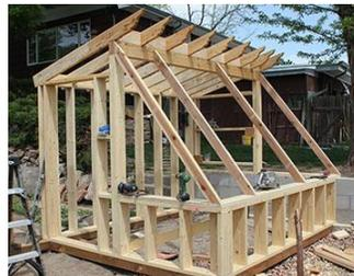
The hobby greenhouse is a 2x6 wood-frame construction, allowing for more insulation.
