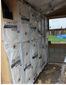
and heat tight. He insulated the framed walls and roof with fiberglass — essential for keeping plants warm during cold winter months.
