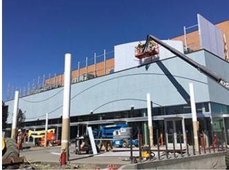
the top to achieve a specific 'flow' and is lit from below. The material specified by the architect was a 16mm 5-wall X-structure panel. Multiwall polycarbonate offers
