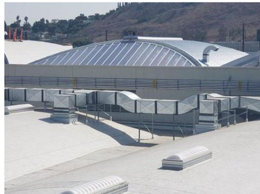
The daylighting system used was Duo-Gard's Series 3600 Sloped Glazing system. Combining natural light, design versatility, and high performance, the three custom skylights that were installed were glazed with 25mm multiwall polycarbonate clear panels.
