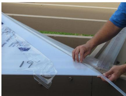
Using polycarbonate U- and H-profiles can help achieve a finished and professional look for your multiwall polycarbonate project. A polycarbonate U-profile is used to cap off the top and
