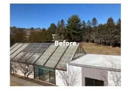
to be replaced. The original glazing was replaced with LEXAN™ THERMOCLEAR™ Plus 25mm 5x-wall clear panels. These high-performance polycarbonate panels fit seamlessly into OpenAire's extrusion system, making the installation process relatively quick and simple.
