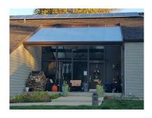
This multiwall polycarbonate product combines high light transmission and good thermal insulation in a lightweight yet durable sheet.
