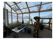
Trevor chose 10mm multiwall polycarbonate as the glazing material for his greenhouse. Translucent polycarbonate panels cover part of the roof, half of the east and west walls, and the entire south-facing wall of the building. The clear multiwall panels allow for maximum light transmission to enter the PSG while the hollow structure offers excellent thermal properties.
