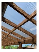
Durable yet lightweight, multiwall polycarbonate is an ideal patio roof covering that is easy to cut, install, and maintain.
