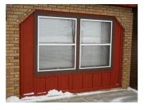
Multiwall polycarbonate can easily be cut to the size or shape of your window and attached to the window frame with self-adhesive
