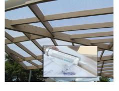
choosing the right one for your project is very important. For polycarbonate sheet applications, it is highly recommended to use a 100% silicone sealant. As the name suggests, a 100% silicone sealant is not 'cut' with any solvents or oils.
