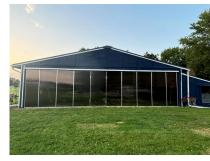
Jason described the installation of the multiwall panels and aluminum profiles as a bit challenging but mostly due to squaring up the existing hangar door. "The aluminum base and cap system worked well, the instructions were good, and Tony Newberry (AmeriLux Experience Specialist) helped me out when I didn't read all the instructions. Once we got the system down, the panel install time was reduced significantly."
